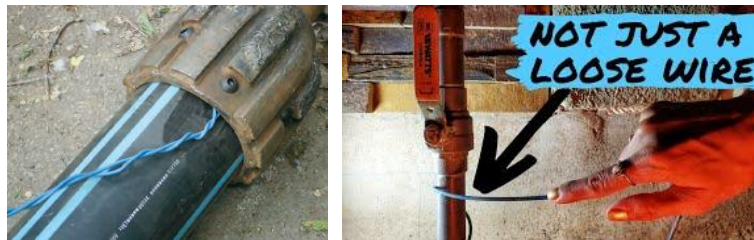
Figure 6 – “Blue” Tracer Wire
