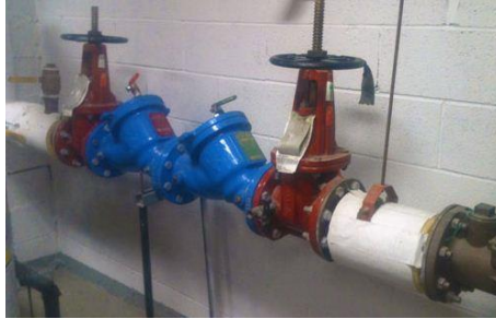
Figure 8 – Example of a Backflow Prevention Assembly
